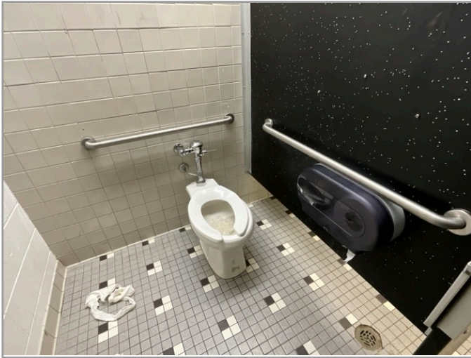
TOILET STALL OVERVIEW
