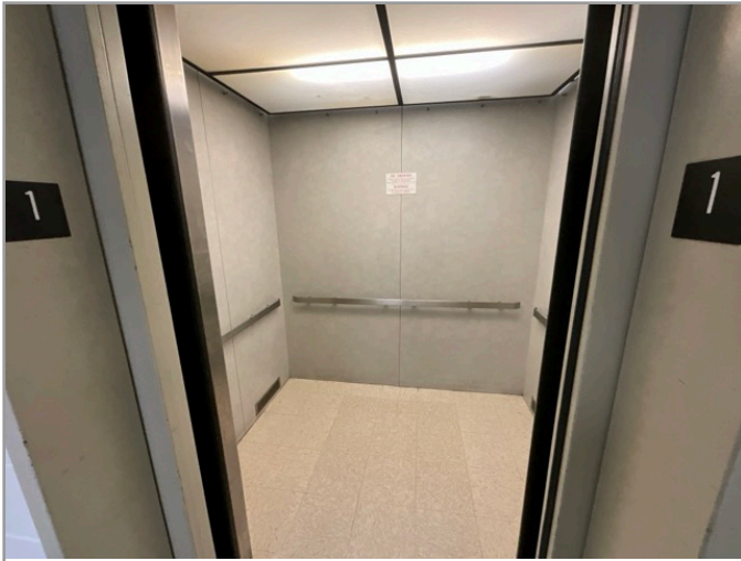
LOBBY LOOKING AT CABS (WITH DOORS OPEN)
