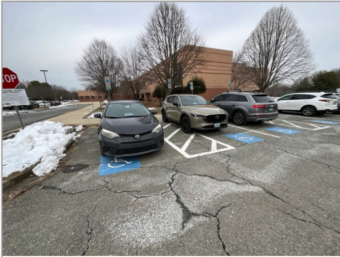
OVERVIEW OF ACCESSIBLE PARKING AREA
